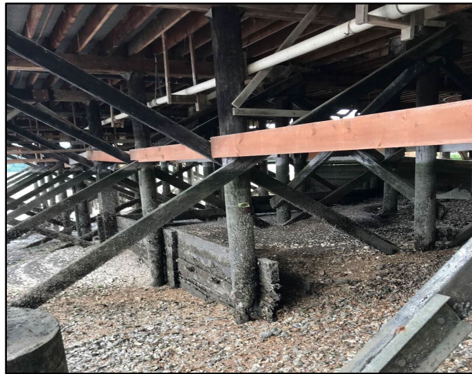
Figure 28: No Removal Credits for Non-Functional Shoreline Armoring that is not in good condition. Removal credits do not apply for horizontal pile stabilizer as there is no functioning bulkhead effect (like sediment retention behind the bulkhead or elimination of water exchange).
